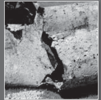
Does your septic system have a steel tank installed before 1970? If so, it may look like these and need replacement. Photos supplied by the Timiskaming Health Unit.
